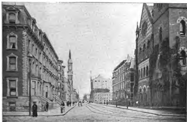
ST. BARTHOLOMEW'S CHURCH. MANHATTAN ATHLETIC CLUB. HOLY TRINITY CHURCH. MADISON AVENUE, LOOKING NORTH FROM 42d STREET.
